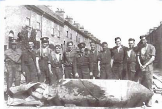
Fredrick Road, Gorleston, June 12th, 1941
